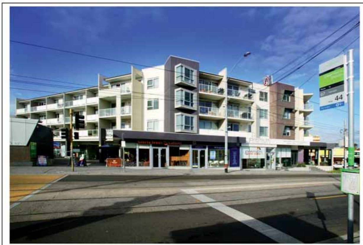
Elsternwick Station: Modernised station with retail and residential mixed development.
